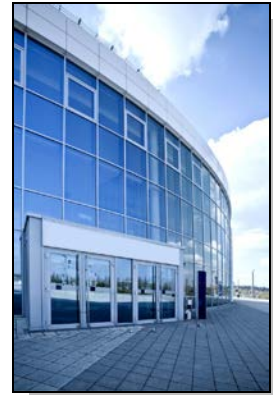
Facilities Information Management System
