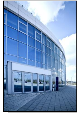
Facilities Information Management System
