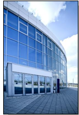
Facilities Information Management System
