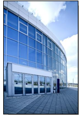
Facilities Information Management System
