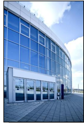
Facilities Information Management System
