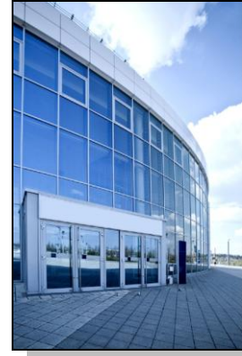
Facilities Information Management System
