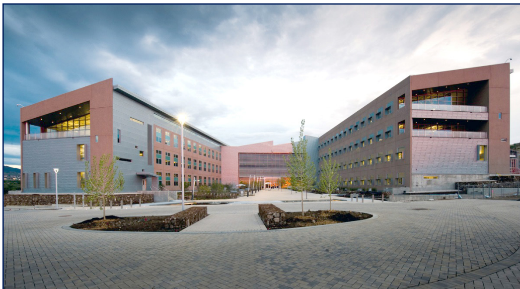
Research Support Facility at the National Renewable Energy Laboratory (NREL). NREL's Research Support Facility, completed in 2010, is a sustainable green building. This 218,000 square foot office building includes a rooftop photovoltaic system, daylighting, natural ventilation, and a next-generation, energy efficient data center.
