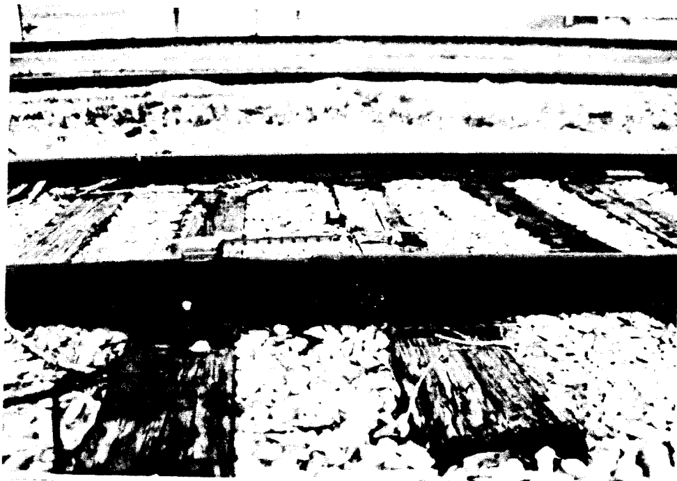
BROKEN RAIL HEAD AT JOINT, LOOSE BOLTS, NON-STANDARD TIE PLATES AND DEFECTIVE TIES
