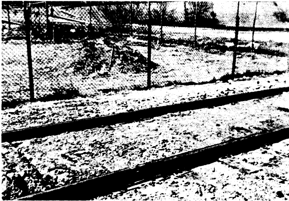
RAIL PULLAPART. NO RAIL ANCHORS AND DEFECTIVE TIES
