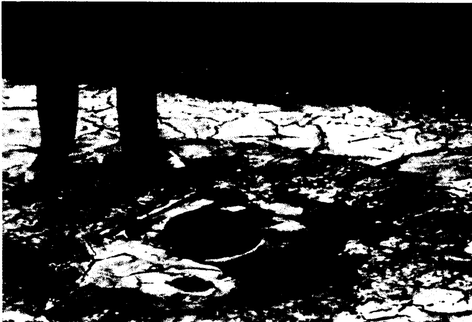
DRAIN NOT LOCATED AT POINT OF MAXIMUM ROOF DECK DEFLECTION
