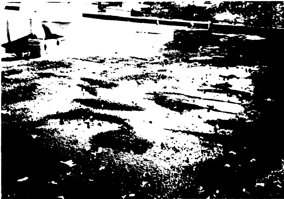
LARGE BLISTERS AND BUCKLES
