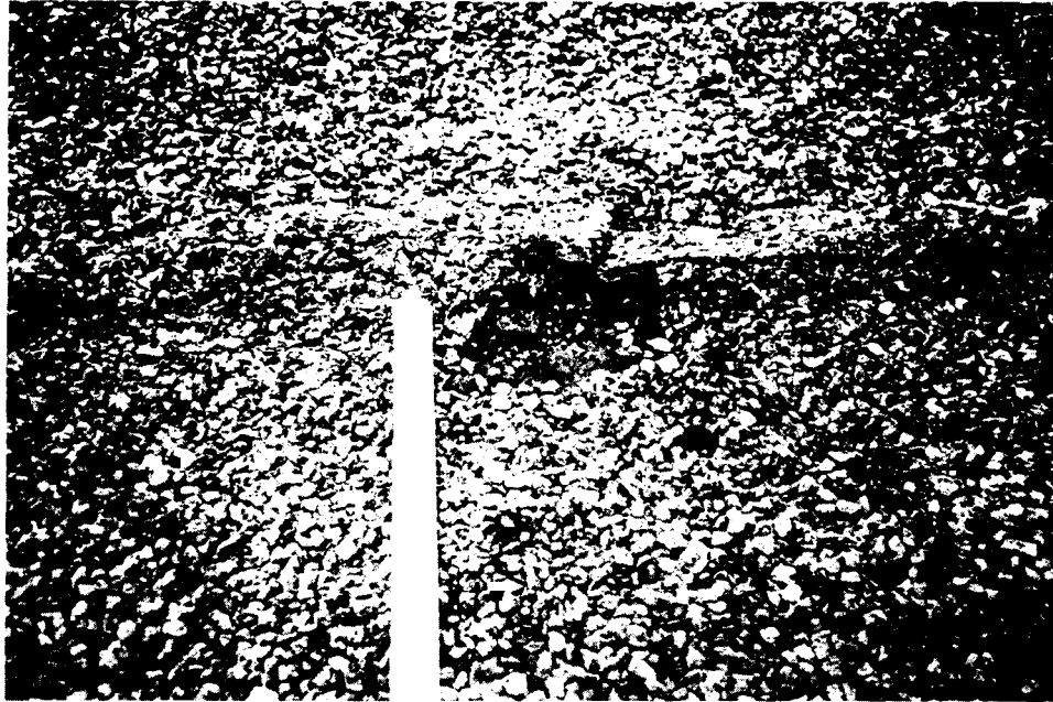
PUNCTURES IN MEMBRANE
