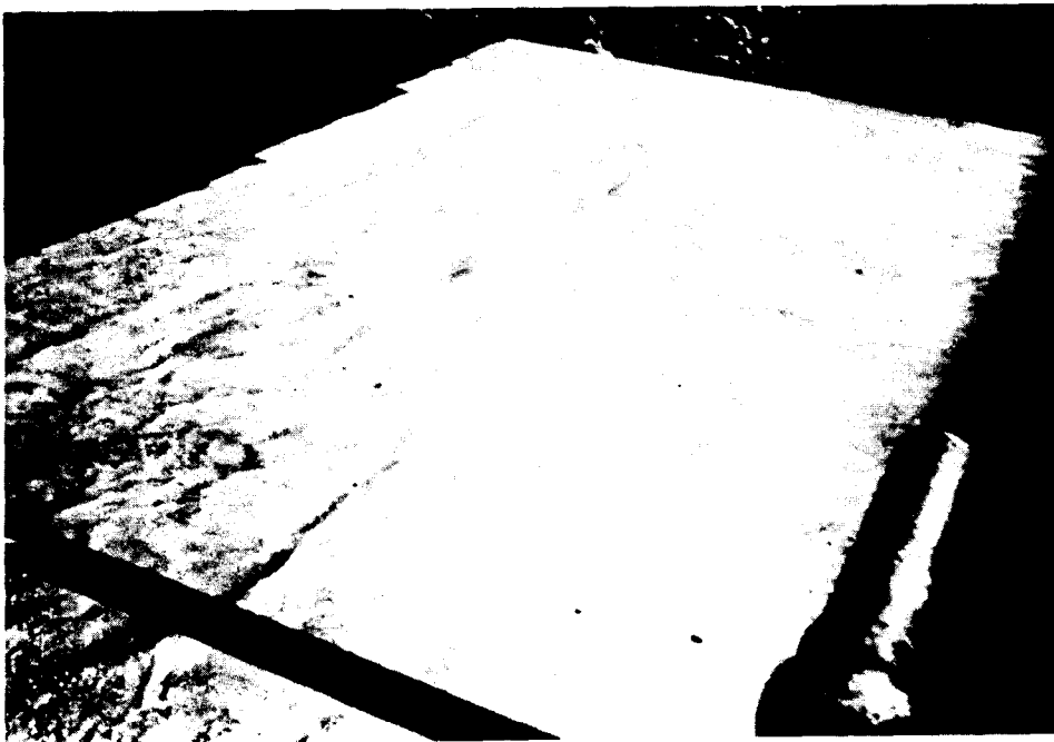
MEMBRANE DELAMINATION
