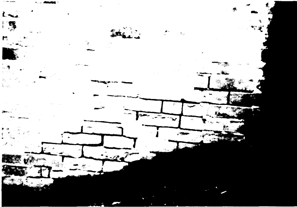
MORTAR JOINTS DETERIORATING
