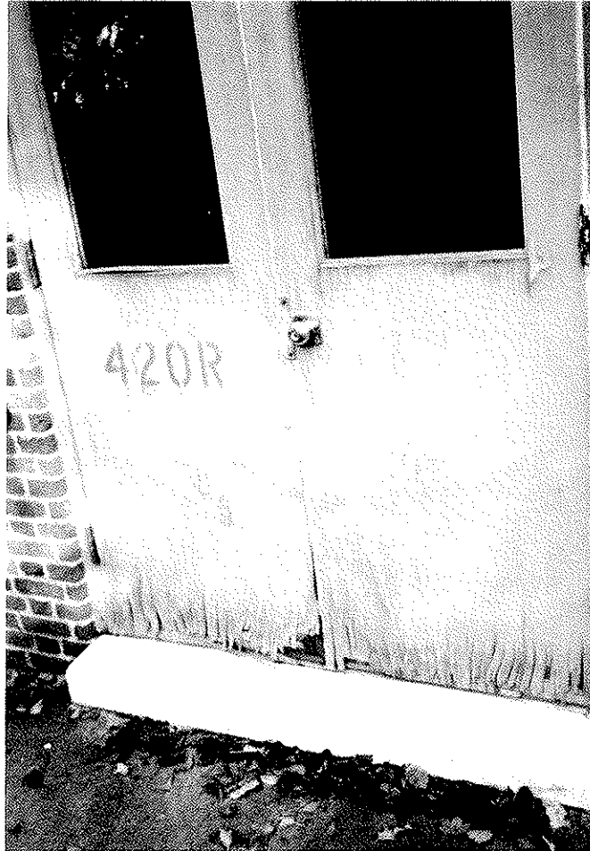
DELAMINATING AND WATER DAMAGED WOOD DOOR
