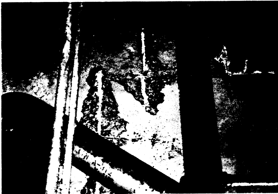
SLAB SPALLING
