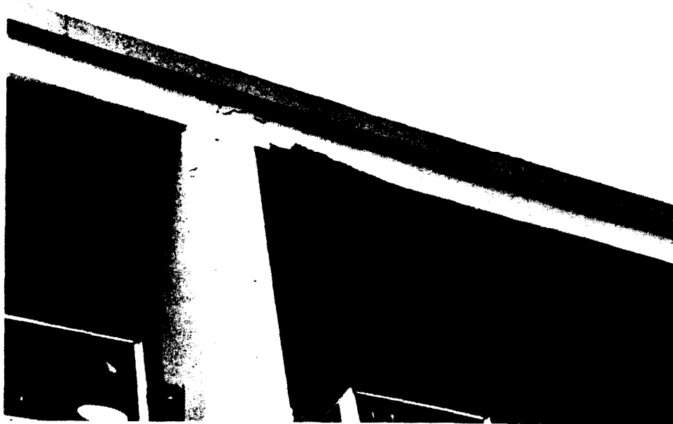
COLUMN CRACKING CAUSED BY FOOTING MOVEMENT
